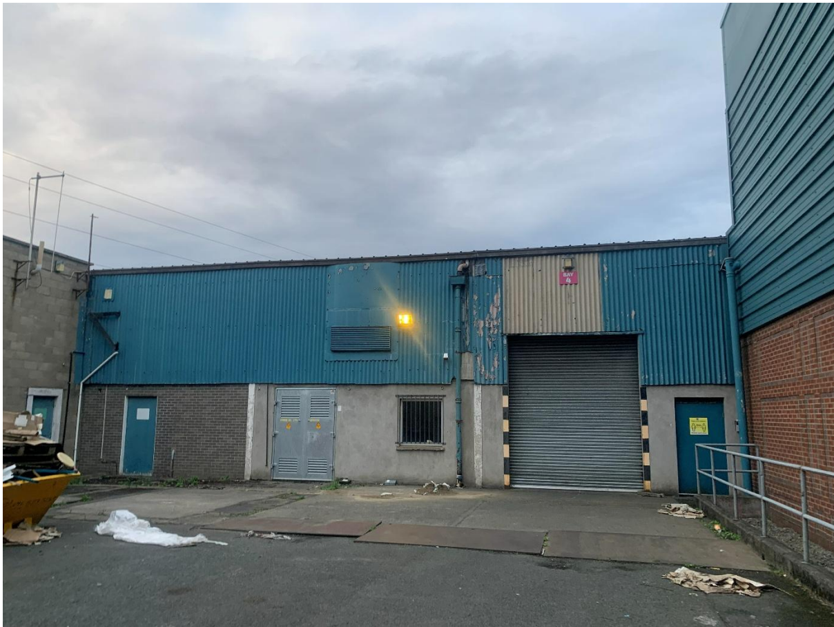
Plate 9. Western loading port at VSDirect warehouse.
