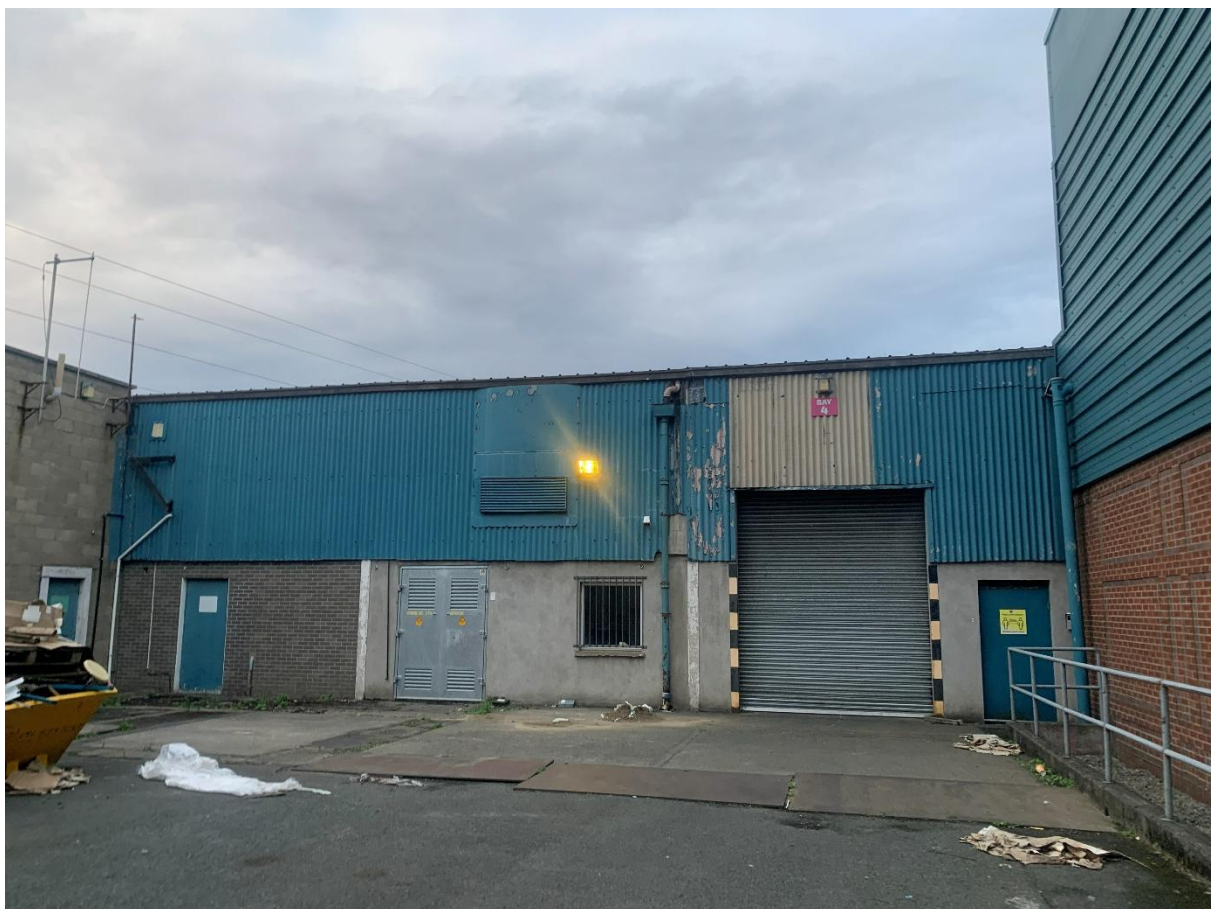
Plate 9. Western loading port at VSDirect warehouse.
