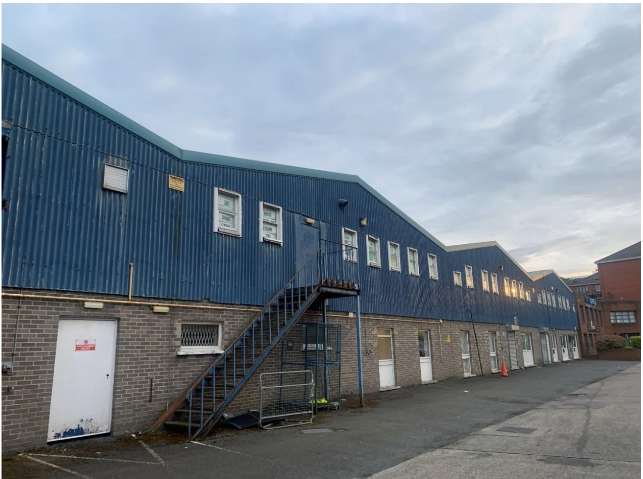
Plate 7. Northern face of VSDirect warehouse.
