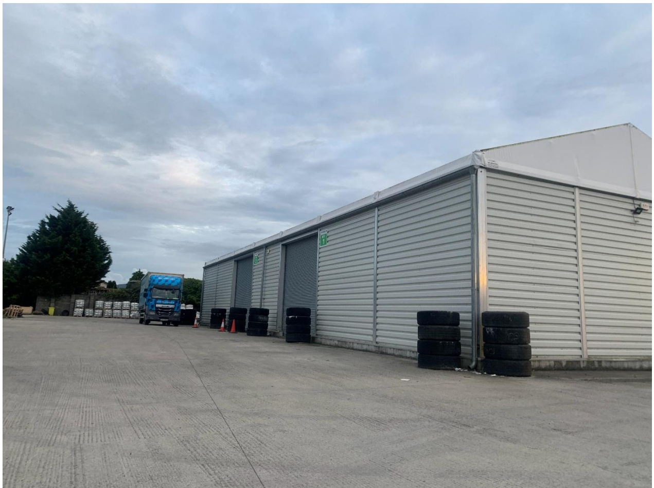
Plate 5. Eastern face of VSDirect warehouse.
