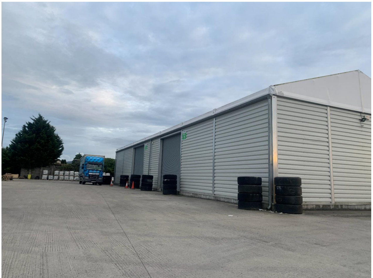
Plate 5. Eastern face of VSDirect warehouse.
