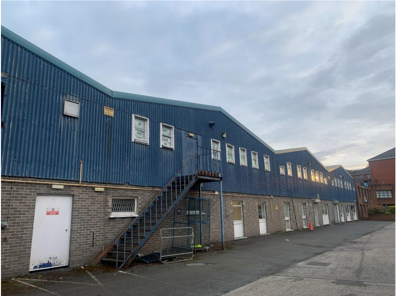
Plate 7. Northern face of VSDirect warehouse.
